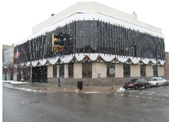
Above is a picture of our new building!
